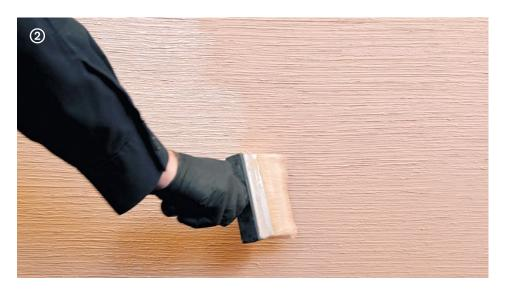
→ Decor must be applied over the whole surface, by brush, in one or two coats, either pure or diluted to a maximum of 5 - 10%, following the direction of the horizontal lines.
