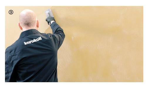
$\rightarrow$  Apply the 2<sup>nd</sup> coat once the material has hardened (3-12 hours). Tip: if crests or flashes are present, sand in order to remove them before applying the 2<sup>nd</sup> coat. A drop of water may be added in order to make the product more workable.
