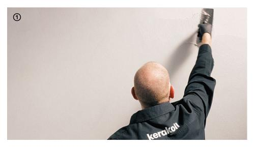
→ Apply the 1st coat of **Wallcrete** spreading the product with small and even strokes of the spreader over the entire surface.
