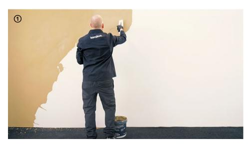
→ Apply the 1st coat of **Patina** spreading the product with small and even strokes of the spreader over the entire surface.
