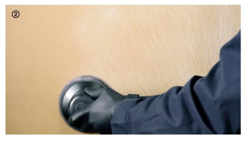
→ After 4-6 hours, sand the surface with 80-120-grain sandpaper in order to remove any small imperfections and to make the surface smooth and pleasing to the touch.
