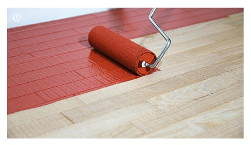
→ Evenly apply the 1<sup>st</sup> coat of **Microresina** with **Roller Plus** respecting the coverage of  $\approx$  110 g/m<sup>2</sup>.
