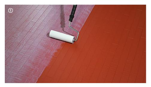
→ Evenly apply Microresina Xtreme with Roller Plus respecting the coverage of ≈ 80 ml/m<sup>2</sup>.
