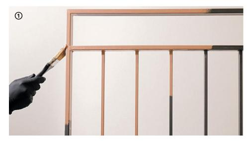
→ On irregular surfaces, Microresina may be applied by brush in two, three or more coats until the required coverage is achieved (according to the colour used).
