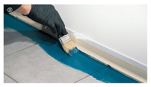
→ Shape the corners with a brush or a small roller as you gradually proceed, so that the product can always be overlaid wet-on-wet.
