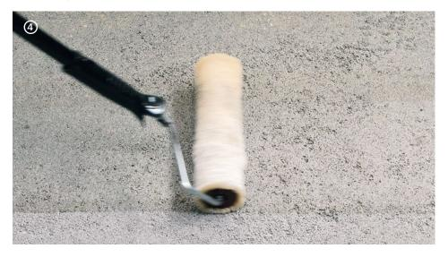
→ The absorbent cement-based substrates must be treated with EP21 applied neat and spread using a roller with a coverage of ≈ 200 ml/m². Tip: flaky substrates must be treated with 2 coats of EP21. The 1st coat diluted with Keragrip Eco Pulep up to 30%, the 2<sup>nd</sup> coat, 6 hours later, with pure EP21.
