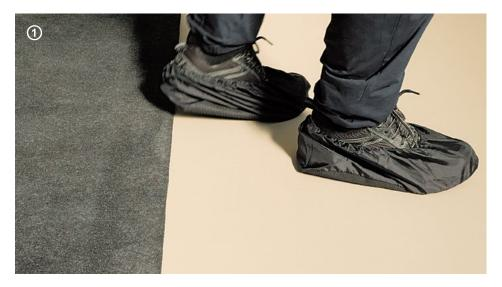
$\rightarrow$  Be careful not to dirt **Cementoresina 2** with any plastic or metallic parts of shoes, knee pads or tools.
