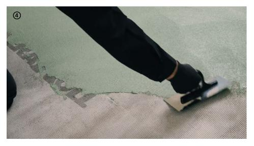
→ Spread the product with a finishing trowel and level to cover the Net
