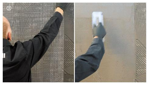
→ Lay the mesh on the product while it is still wet and overlap it with the one next to it for 10 cm; then smooth with a smooth spreader, level to cover the **Net 90** fibreglass reinforcing mesh and remove any excess.
