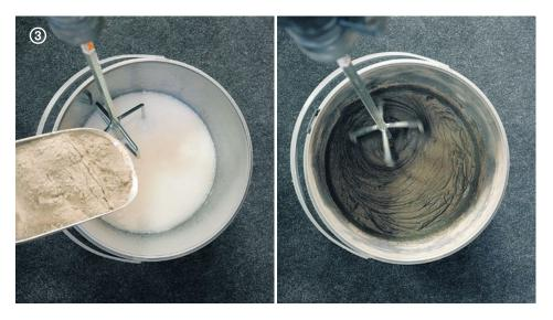
→ Wallzero is prepared by mixing together parts A and B, respecting the mixing ratio A : B = 100 : 14. Add water until the required consistency is reached ≈ 3 I / 1 bag (25 kg).
