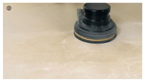
→ Sand the **Cementoresina 2** layer with a floor buffer (120 grain) and thoroughly vacuum to remove sanding residues.
