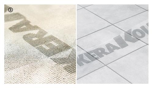
$\rightarrow$  Spread the **Net 90** fibreglass reinforcing mesh on the whole surface, bringing the edges of the mesh together.
