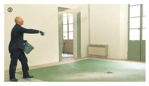
→ Sprinkle wet on wet to saturation with **Quarzo 1.3** maintaining the coverage of  $\approx 2 \text{ kg/m}^2$ .
