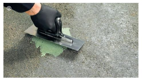
→ Before applying on the whole flooring, if need be a local preliminary grouting may be carried out in order to repair small, few-millimetre-thick imperfections of the substrate.
