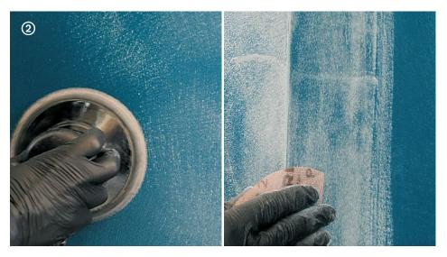
→ If any visible crests or accumulation of material form at the corners when applying the 1<sup>st</sup> coat of **Cementoresina Wal**, they must be removed by using the trowel blade or a grade 60 sandpaper, either by hand or using a sander.
