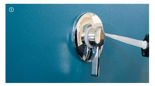
→ After the application, use Tetra Fix Crystal sealant or Silicone Color to seal plaques, vents, shower cabinets and drains in environments with frequent contact with water.
