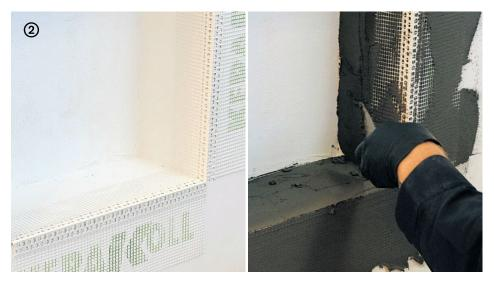
→ Use straight, rigid PVC or aluminium corner pieces to reinforce the edges when it is necessary to incorporate edge beads into Wallzero in showers, bathtubs, Turkish baths, washbasin recesses or counters.
