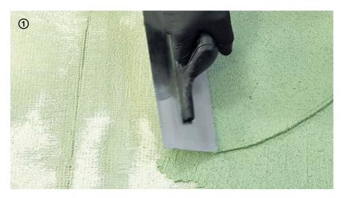
→ In case of a particularly irregular substrate, or in case of deep joints, apply a  $2^{nd}$  coat of **Floorzero** in order to perfectly level the surface.
