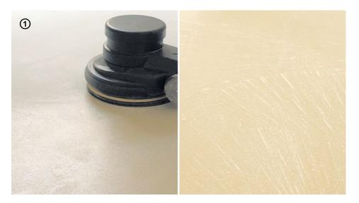
→ Sand the **Cementoresina** 1 layer with a floor buffer (120 grain) and thoroughly vacuum to remove sanding residues.
