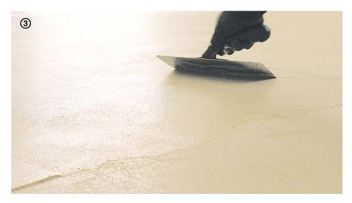
→ Smooth the product on the floor using small semi-circular movements of the trowel without leaving crests or ridges. The trowel must slide over the preceding layer so that the product is completely smoothed off.
