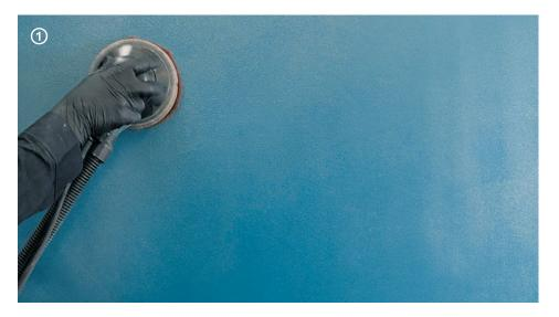
→ Sand Cementoresina Gel with a rotating orbital sander with Softpad felt disk. Vacuum thoroughly to remove sanding residue.
