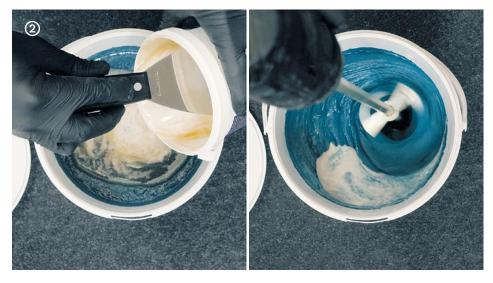
→ Pour part B following the catalysis ratio A : B = 3 : 0.4. After carefully mixing with a helicoidal agitator for the first time, run a scraper along the sides and bottom of the bucket to mix all parts left unmixed by the agitator. After cleaning the scraper, mix again.
