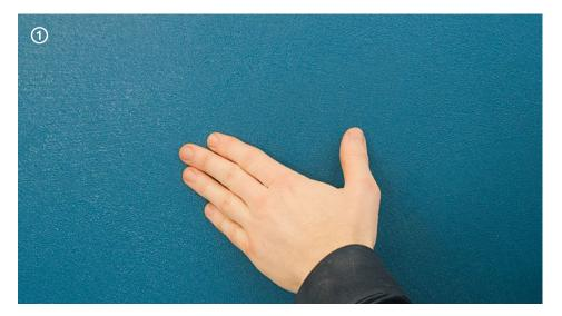
→ When applied as 1<sup>st</sup> coat, Cementoresina Wall can be overlaid after 14 hours from its initial application. The layer can be overlaid even if it is still "tacky" on the surface.
