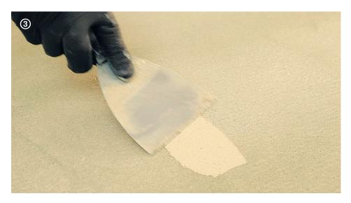
→ Before the application check that Floorzero has no defects and imperfections and that the Net 90 mesh is not showing.
