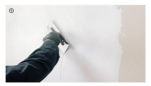
→ Apply the 1st coat of **Wallpaper** spreading the product on the surface in order to even and level it.
