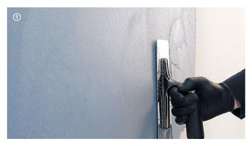
→ Apply the 1<sup>st</sup> coat of **Patina** spreading the product with small and even strokes of the spreader over the entire surface.
