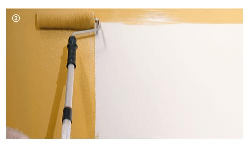
→ **Microresina** must be carefully applied with a roller over the whole surface in two-three coats, diluted to a maximum of 10%.
