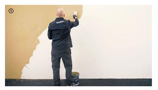
$\rightarrow$  Apply the 1<sup>st</sup> coat of **Patina** smoothing the product with small and even strokes of the spreader over the entire surface.
