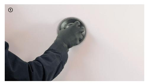
→ Before applying **Decor**, sand the surface with 80 - 220-grain sandpaper in order to make the surface perfectly smooth and pleasing to the touch.
