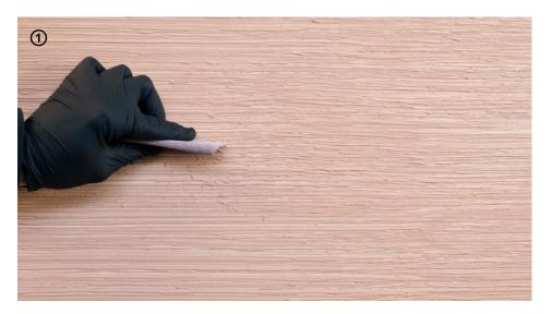
→ Lightly sand by hand in order to remove any small flaws or lumps before applying **Decor**.
