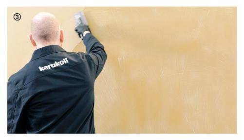
→ Apply the  $2^{nd}$  coat once the material has hardened (3 - 12 hrs). Tip: if crests or flashes are present, sand in order to remove them before applying the  $2^{nd}$  coat. A drop of water may be added in order to make the product more workable.
