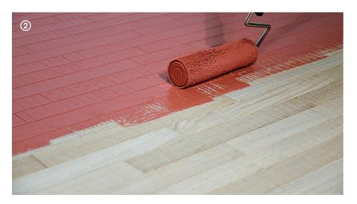
Tip: apply first the product in one direction and then in the other, in order to obtain a complete and even coverage of both the texture and the chamfer.
