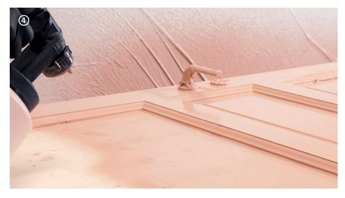
Tip: be careful not to overload the surface in order to avoid drips or droplets.
