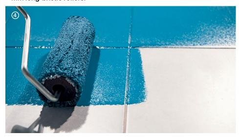
Tip: carefully and evenly apply the product in the joints as well. In joint areas, blend together by lifting up the roller, in order not to leave excess amounts of material.
