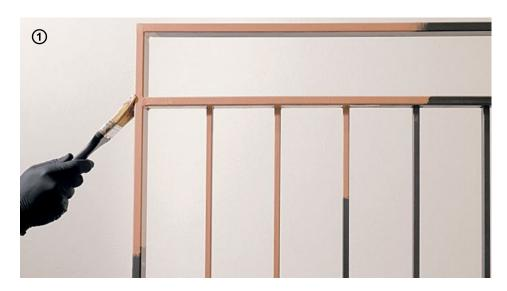
→ On irregular surfaces, Microresina may be applied by brush in two, three or more coats until the required coverage is achieved (according to the colour used).
