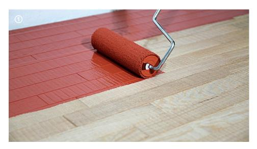
$\rightarrow$  Evenly apply the 1st coat of **Microresina** with **Roller Plus** respecting the coverage of  $\approx$  110 g/m<sup>2</sup>.
