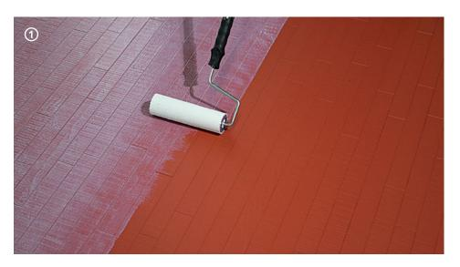
$\rightarrow$  Evenly apply **Microresina Xtreme** with **Roller Plus** respecting the coverage of  $\approx$  80 ml/m<sup>2</sup>.
