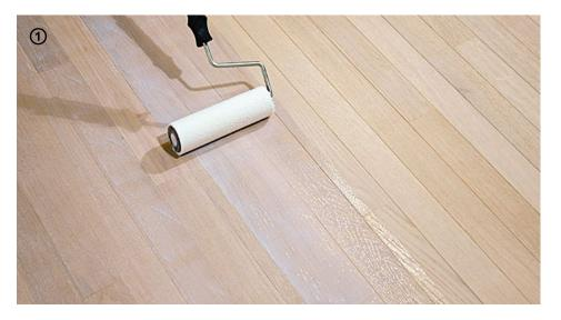
→ Evenly apply three coats of **Microresina Xtreme** with **Roller Plus** respecting the coverage of  $\approx 80$  ml/m<sup>2</sup>.
