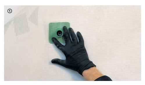
$\rightarrow$  First prepare the layers of **Net 90** mesh, cutting it where needed.
