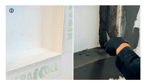
→ Use straight, rigid PVC or aluminium corner pieces to reinforce the edges when it is necessary to incorporate edge beads into Wallzero in showers, bathtubs, Turkish baths, washbasin recesses or counters. Tip: we recommend using PVC edge beads.
