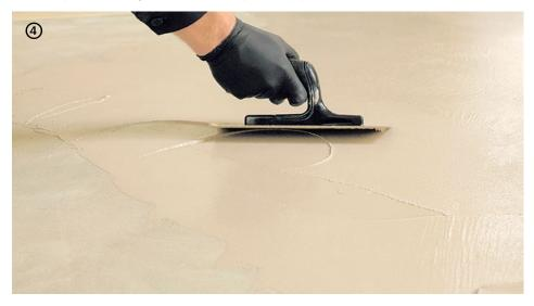
→ Smooth the product on the **Floorzero** support layer using small semicircular movements of the trowel without leaving crests or ridges.
