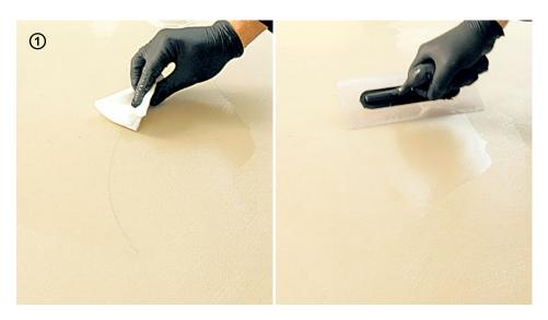
→ In case of stains or marks when applying **Cementoresina Gel**, clean with a cloth soaked in **Keragrip Eco Pulep**; then apply again **Cementoresina Gel** in the same spot and proceed with the application.
