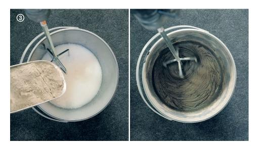
→ Wallzero is prepared by mixing together parts A and B, respecting the mixing ratio A : B = 100 : 14. Add water until the required consistency is reached ≈ 3 I / 1 bag (25 kg).
