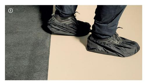
→ Be careful not to dirt **Cementoresina 2** with any plastic or metallic parts of shoes, knee pads or tools.
