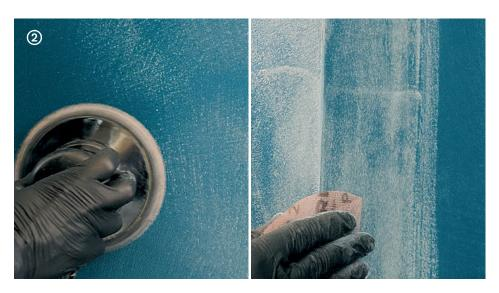
→ If any visible crests or accumulation of material form at the corners when applying the 1st coat of **Cementoresina Wall**, they must be removed by using the trowel blade or a grade 60 sandpaper, either by hand or using a sander.
