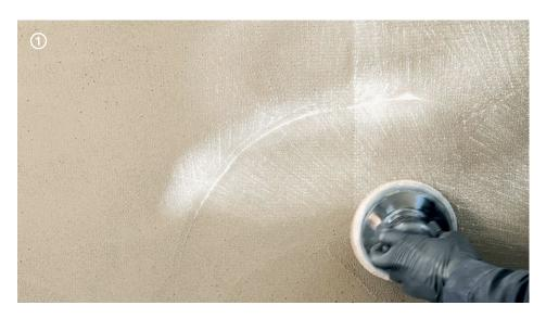
→ Before the application, check that Wallzero is perfectly levelled, that imperfections of the substrate have been covered and removed, and that the Net 90 mesh is not showing. Sand Wallzero with a rotating orbital sander (40 grain) and clean any sanding residue.
