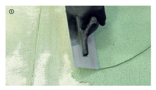
$\rightarrow$  In case of a particularly irregular substrate, or in case of deep joints, apply a 2<sup>nd</sup> coat of **Floorzero** in order to perfectly level the surface.
