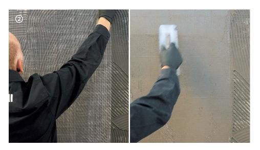
→ Lay the mesh on the product while it is still wet and overlap it with the one next to it for 10 cm; then smooth with a finishing trowel, level to cover the **Net 90** fibreglass reinforcing mesh and remove any excess.
