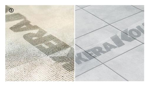
→ Spread the **Net 90** fibreglass reinforcing mesh on the whole surface, bringing the edges of the mesh together.
