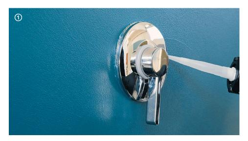
→ After the application, use **Hyperflex Hybrid** clear transparent sealant or **Silicone Color** to seal plaques, vents, shower cabinets and drains in environments with frequent contact with water.
