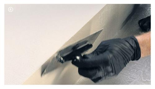
→ On steps, finish the product being careful to cover the corner leaving a small excess of product that will be removed by subsequent sanding.
