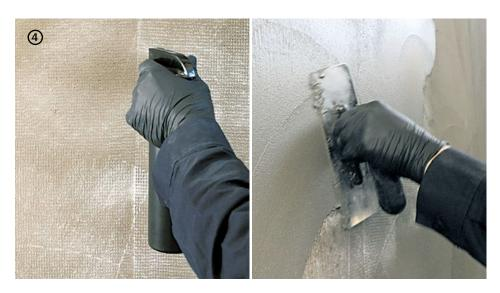
→ After ≈ 3 hours, dampen the 1<sup>st</sup> coat of **Wallzero**, then apply a second coat smoothing the product with small strokes of the trowel in order to obtain a flat and even surface.
