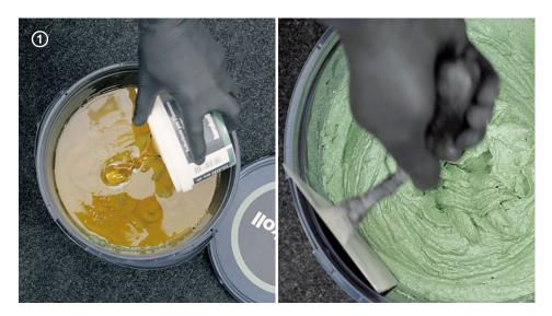
→ Pour part B into the bucket of part A respecting the mixing ratio 9.25 : 0.75. After carefully mixing for the first time with a helicoidal agitator, run a square-sided trowel along the sides and bottom of the bucket, then mix again.
