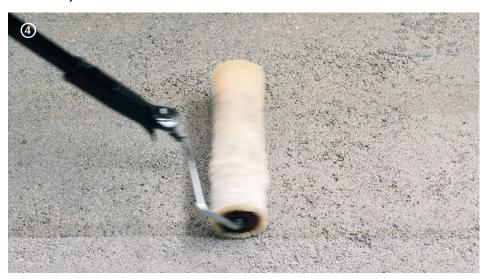
→ The absorbent cement-based substrates must be treated with EP21 applied neat and spread using a roller with a coverage of ≈ 200 ml/m². Tip: flaky substrates must be treated with 2 coats of EP21. The 1st coat diluted with Keragrip Eco Pulep up to 30%, the 2nd coat, 6 hours later, with pure EP21.
