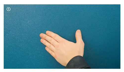
→ When applied as 1<sup>st</sup> coat, **Cementoresina Wall** can be overlaid after 14 hours from its initial application. The layer can be overlaid even if it is still "tacky" on the surface.
