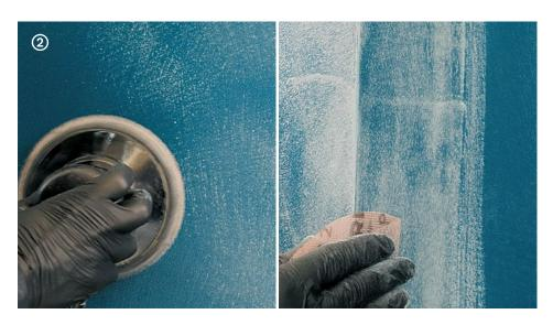
→ If any visible crests or accumulation of material form at the corners when applying the 1<sup>st</sup> coat of **Cementoresina Wall**, they must be removed by using the trowel blade or a grade 60 sandpaper, either by hand or using a sander.
