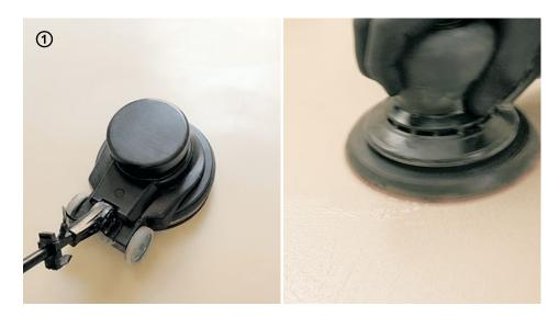
→ Sand **Cementoresina Gel** with a mechanical buffer with **Softpad** felt pad, and thoroughly vacuum to remove sanding residue.
