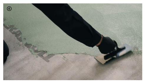
→ Spread the product with a finishing trowel and level to cover the **Net 90** mesh, respecting the coverage of ≈ 2.5 kg/m². Pay attention during application to the complete coverage of the glass fibre mesh.
