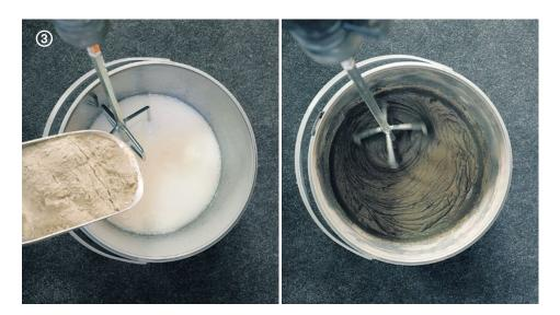
→ Wallzero is prepared by mixing together parts A and B, respecting the mixing ratio A: B = 100: 14. Add water until the required consistency is reached ≈ 3 l / 1 bag (25 kg).
