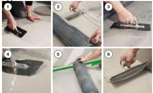
Apply Aquastop Nanoflex with a smooth spreader in thicknesses of about 1 – 2 mm, pressing down to ensure maximum adhesion to the substrate. The resulting thickness depends on the surface finish and on the irregularity of the substrate.
