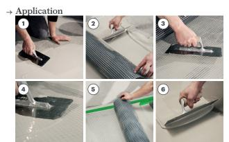
1 Apply Aquastop Nanoflex with a smooth spreader in thicknesses of about 1 – 2 mm, pressing down to ensure maximum adhesion to the substrate. The resulting thickness depends on the surface finish and on the irregularity of the substrate.
