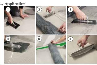
1 Apply Aquastop Nanoflex with a smooth spreader in thicknesses of about 1 – 2 mm, pressing down to ensure maximum adhesion to the substrate. The resulting thickness depends on the surface finish and on the irregularity of the substrate.
